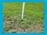
Problem: Poor distribution pattern (brown or dry patches in lawn) <u>Fix</u>: Check nozzle for damage or blockage; replace nozzle with proper pattern; increase or decrease throw distance (distance the water travels out of the spray head) by turning the screw on top of nozzle. Tighten the screw to decrease the throw or loosen the screw to lengthen the distance of the throw.
